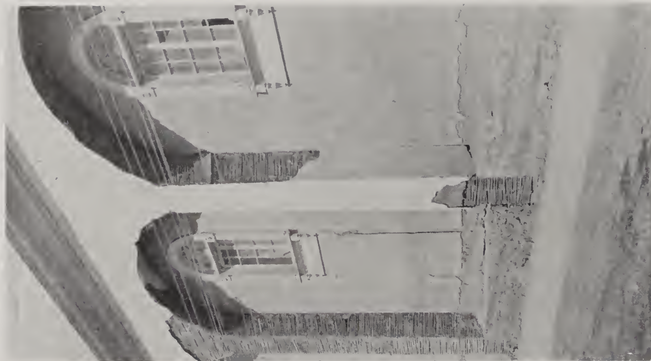
B. Vallenar. Walls of church, showing columns and walls of caña de Guayaquil on frame construction.
