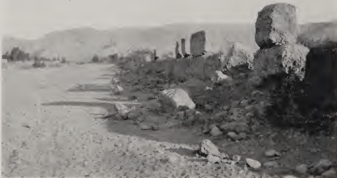
A. Copiapo valley, above Copiapó near Tierra Amarilla. Showing standing and fallen tapiales ; looking south parallel to longitudinal earthquake waves.
