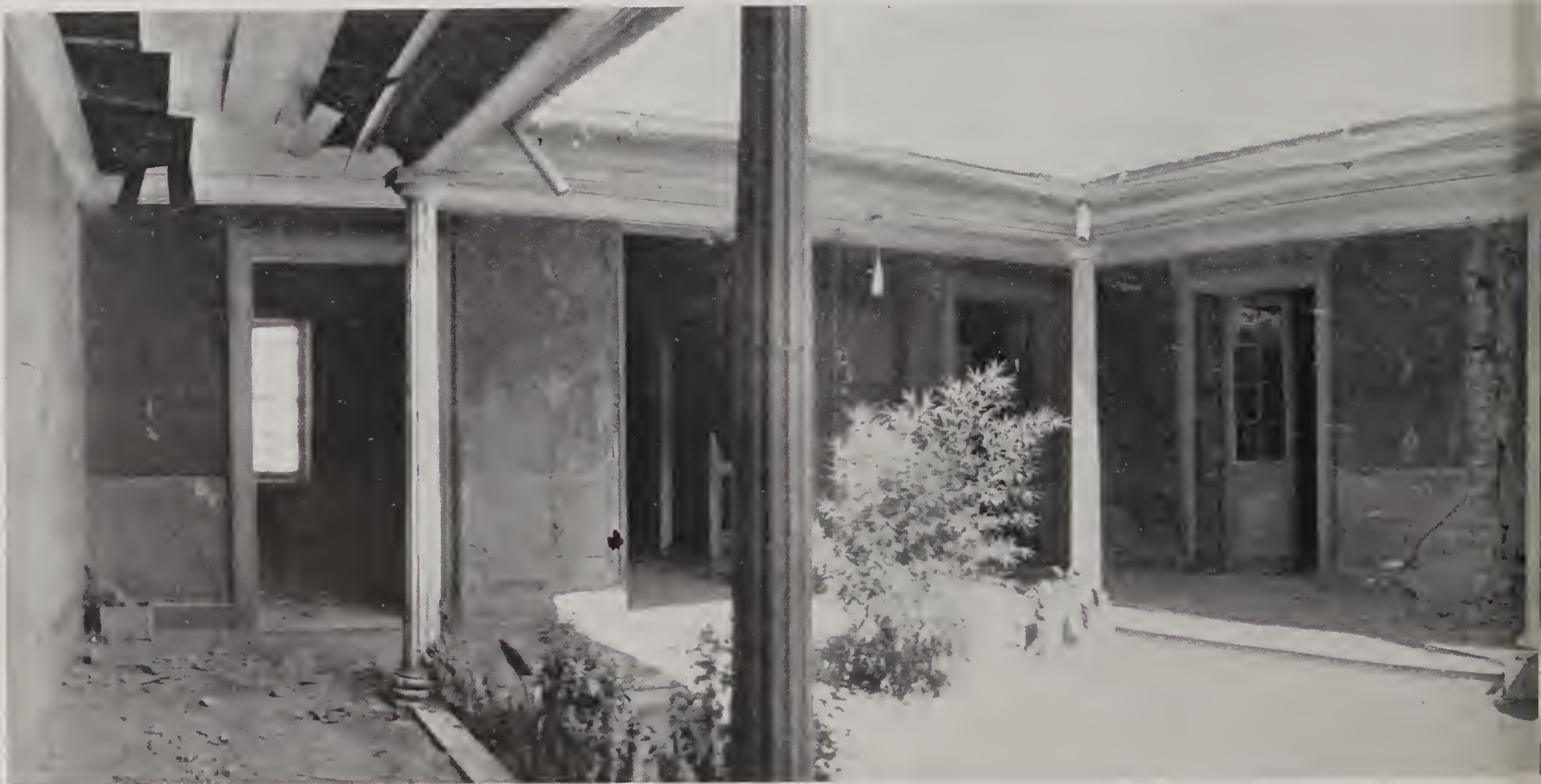
B. Copiapó. Adobe house of one story with light roof, built around a square patio, showing shearing
