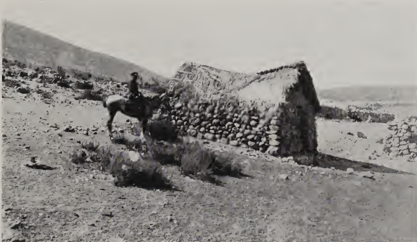
A. Near Coquimbo. Hut, on coast 16 miles (25 km.) south of city, not damaged by earthquake, showing weakness of shock at this point.
