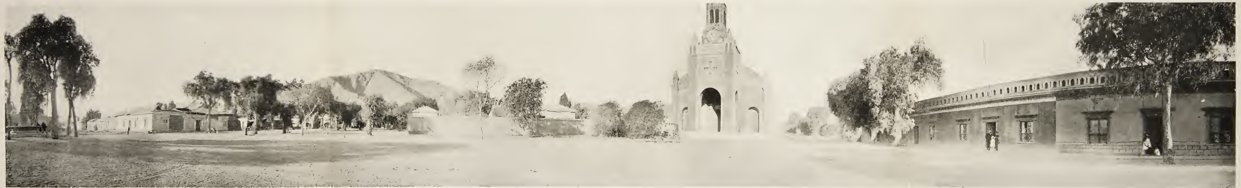
B. Copiapó. Plaza of Juan Godoy. Houses adjoining the plaza on both sides and the church escaped serious damage to their external walls, but interior plastering was generally destroyed. Foundation material is of gravel and construction of buildings is superior to that of most houses in the city. Block of adobe houses on right was built after earthquake in 1810, at a time when necessity for good workmanship was appreciated.
