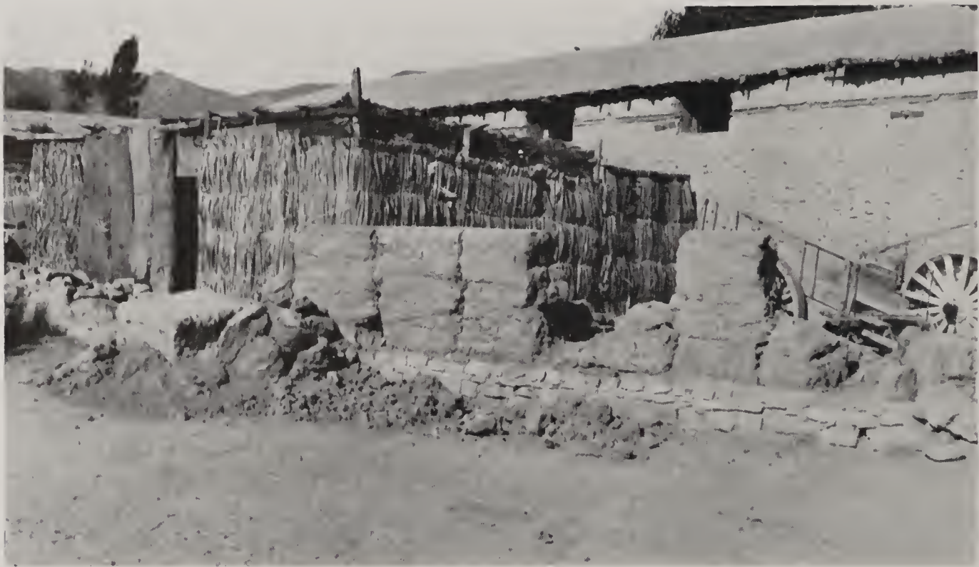
A. Copiapó. Adobe wall of large building intact, tied with timbers; tapiales thrown down, temporary shelter of rushes.
