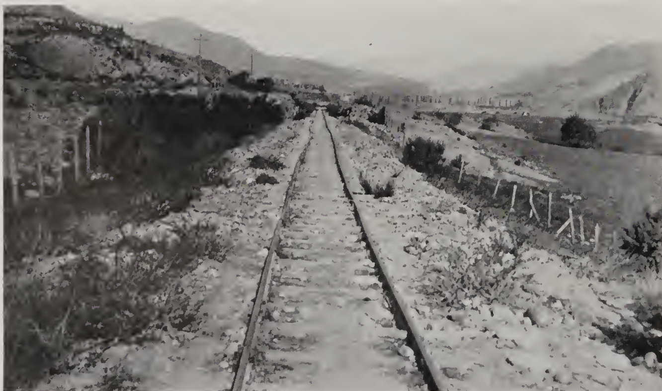
B. Vallenar. Railroad up Huasco valley, showing displacement of track.
