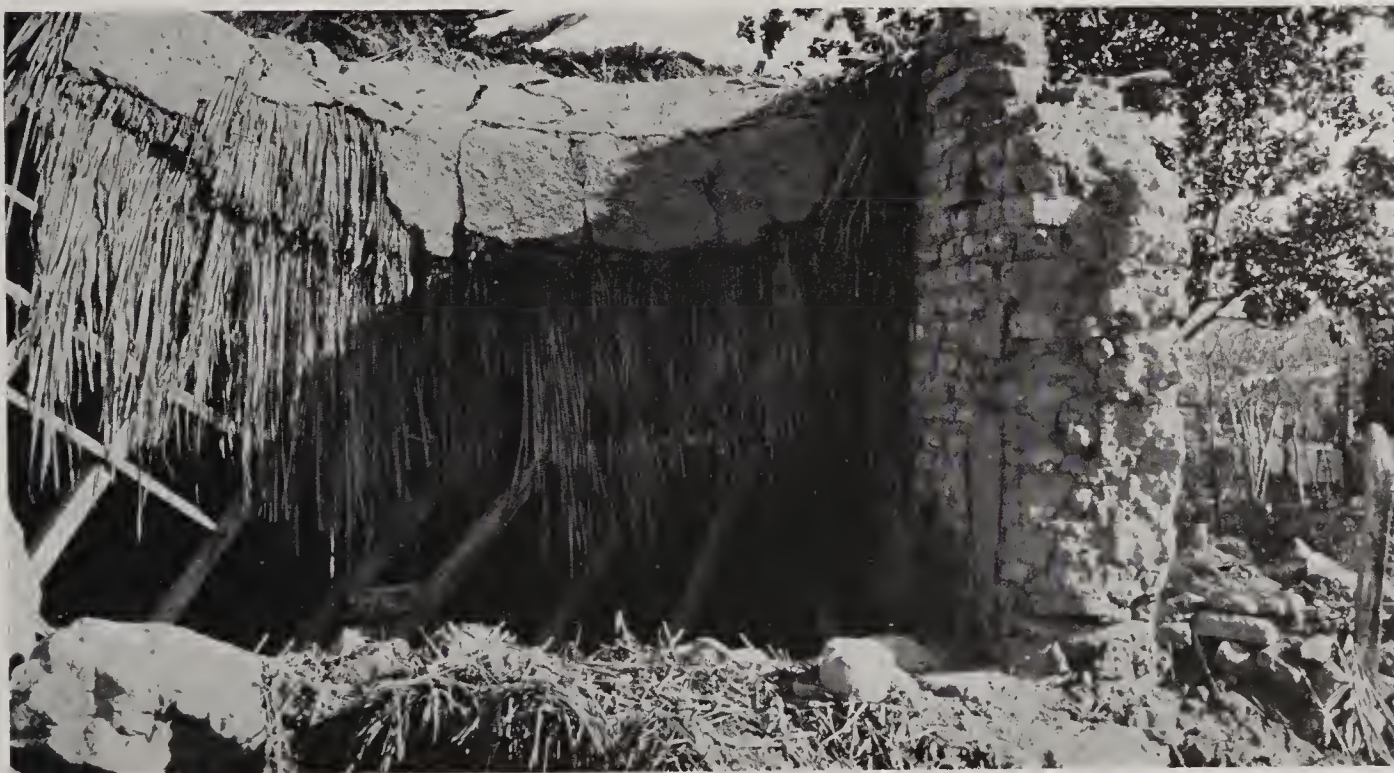
B. Vallenar. Typical ruin of adobe house with heavy mud-covered roof; front wall pushed out by rafters.
