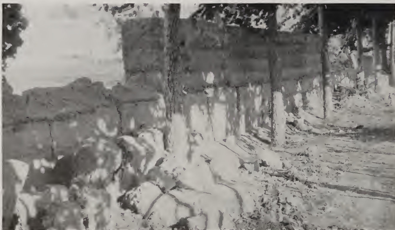
B. Copiapó valley, below Copiapó at Ramadillas. Showing wall of tapiales running N.-S. parallel to longitudinal earthquake waves.
