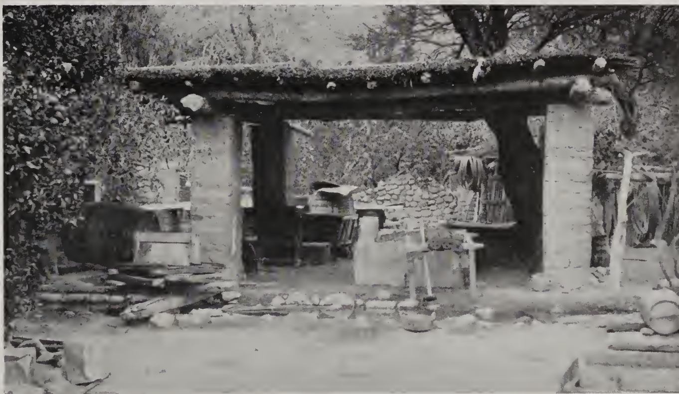
B. La Pampa on Rio Elqui. Columns and roof free to sway but not overthrown.
