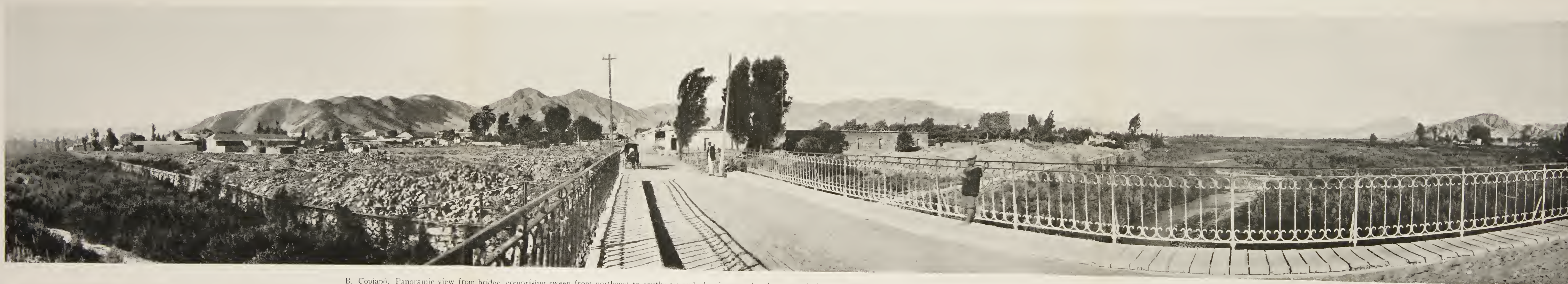
B. Copiapó. Panoramic view from bridge, comprising sweep from northeast to southwest and showing marshy character of river bed. Wall along river bounds area that has been filled in and on which maximum destruction occurred.
