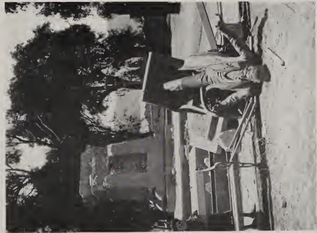
A. Copiapó. Overthrow of Matti monument by failure of pedestal.
