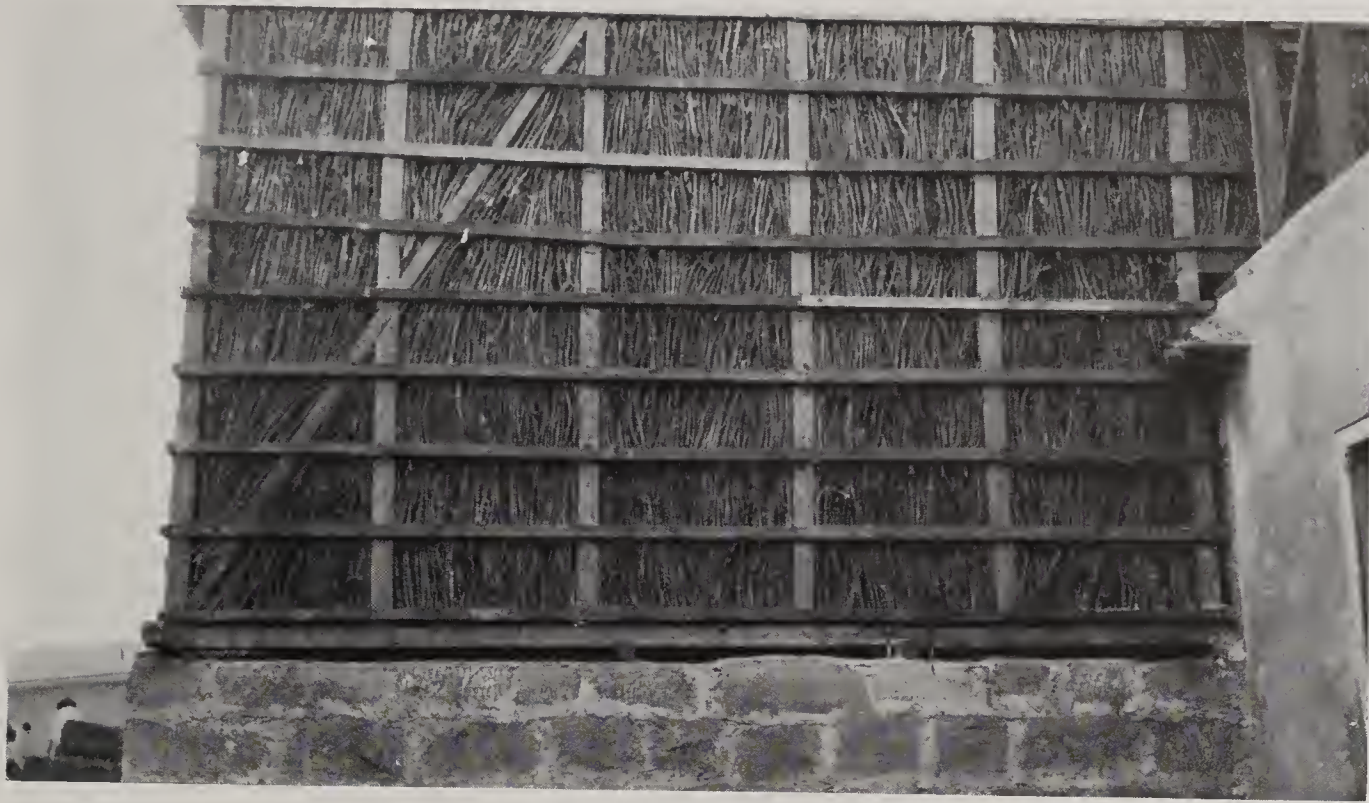
A. First class construction of frame and "brea" or brush; to be plastered with mud.
