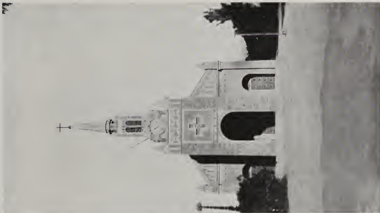
A. Copiapó Church in Plaza Godoy. Frame structure, interior walls and plaster crushed.
