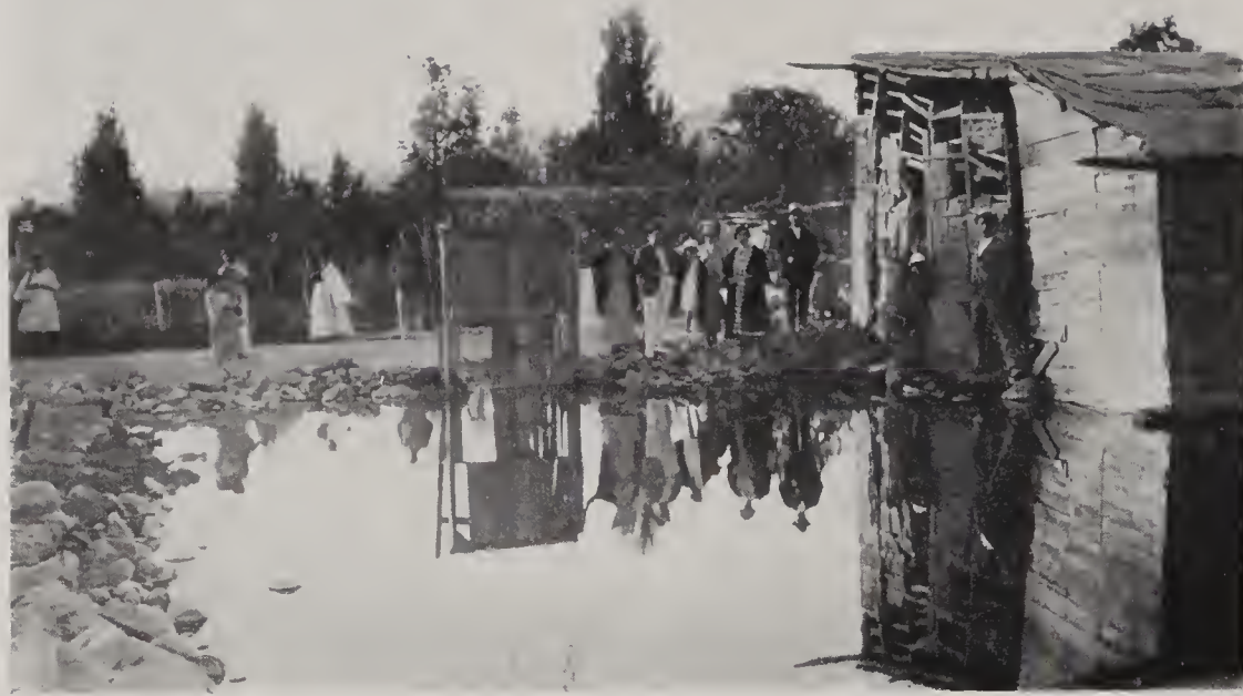
A. Vallenar. Water forced out of river bed by shaking down of alluvium.
