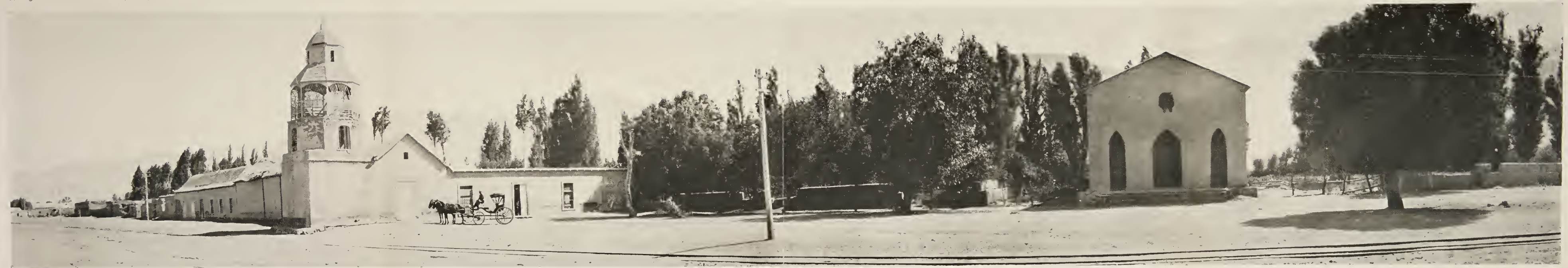
A. Copiapó. The Capella de Candelaria, an adobe chapel more than 100 years old, which has survived repeated earthquakes. Its adobe walls are tied together by iron rods which go through from side to side and are fastened with key plates. The tower is a very light construction with wood frame. On right is a new church built in 1923, collapse of roof of old chapel having rendered it unfit for service.
