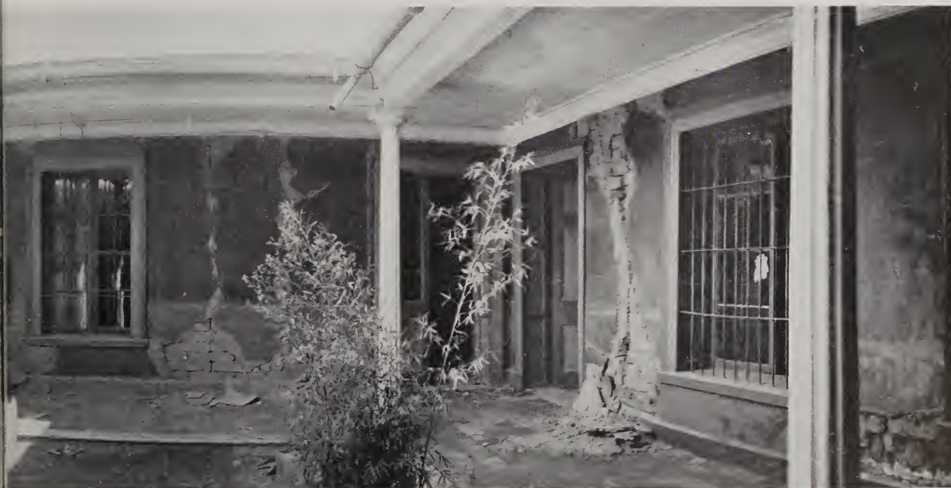
o walls on vertical lines. House was rendered uninhabitable by general fall of plaster walls and ceiling.
