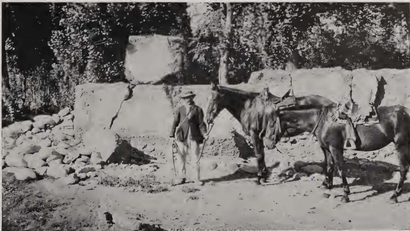
A. Vallenar. Wall of tapiales; two high, partly thrown.
