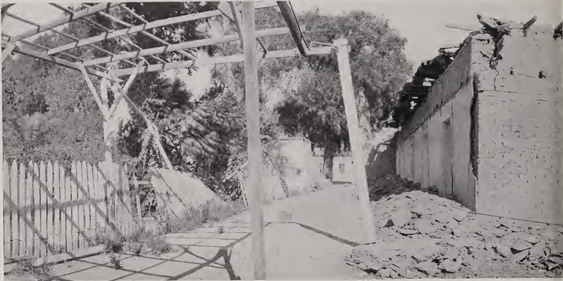
A. Copiapó. Adobe house 70 years old, wrecked by collapse of roof: outer walls suffered but little, being held together by beams.
