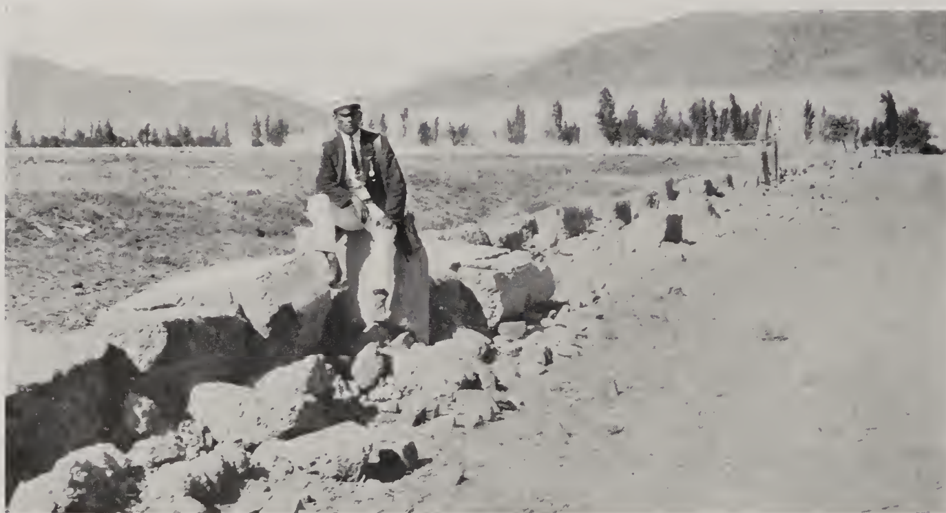
B. Copiapó. General view of tapiale wall running NW.-SE. and of distant wall at right angles to it, showing effect of earthquake.
