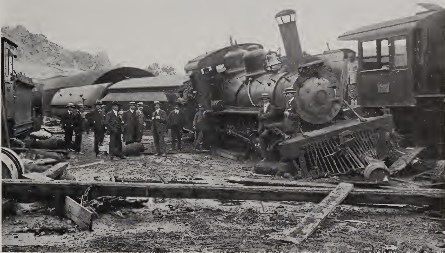
A. Coquimbo. Effects of earthquake wave in railroad yard; height of wave 26 feet (8 meters) above mean tide.
