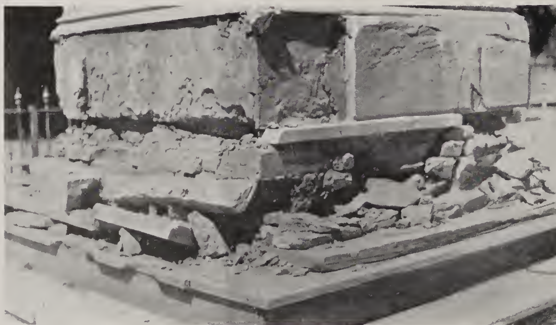
B. Copiapó. Base of Atacama monument, showing detail of brick layer sheared by rotation of upper structure.
