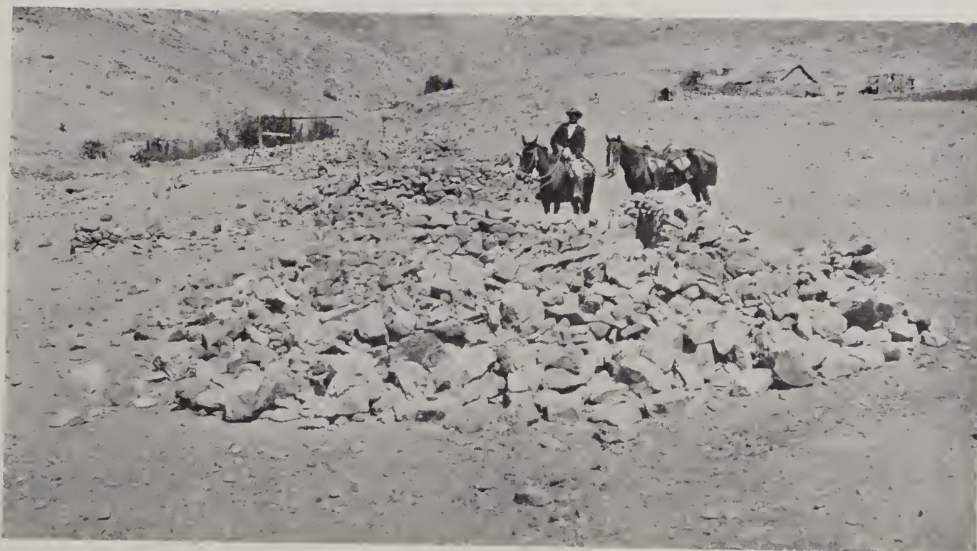
A and B. Vallenar (12.5 miles (20 km.) southwest of). Examples of effect of the earthquake upon massive structures of dry stone walls; located on gravel plain above fault.
