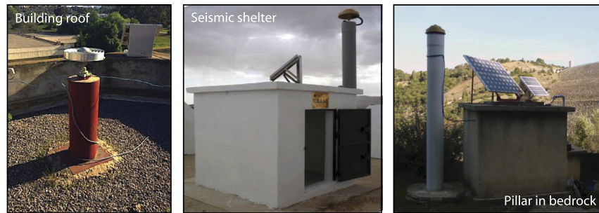
Figure 4. Types of monuments used in the REGAT network. Left: building roof, middle: seismic station shelter, right: 1.5 m–tall concrete pillar anchored in bedrock.
