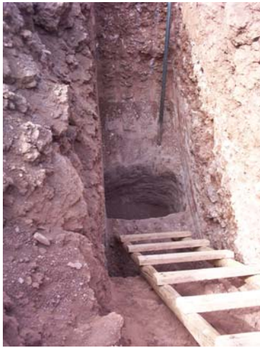
Excavation size : 40x40, 3m depth
