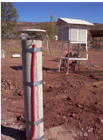
Pillar and receiver shelter
