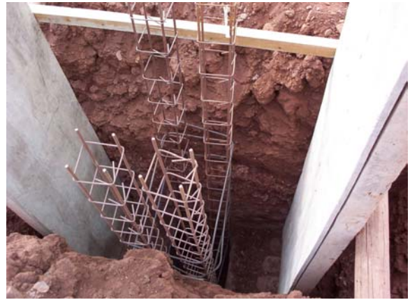
4 10x10 iron stem to re-enforce concrete
