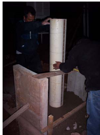
Pilar 1.5m height anchored at 3 m depth
