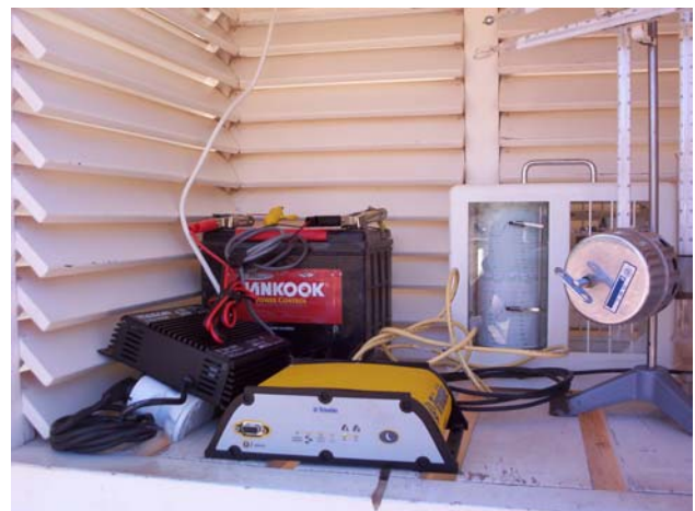
System in meteo shelter
