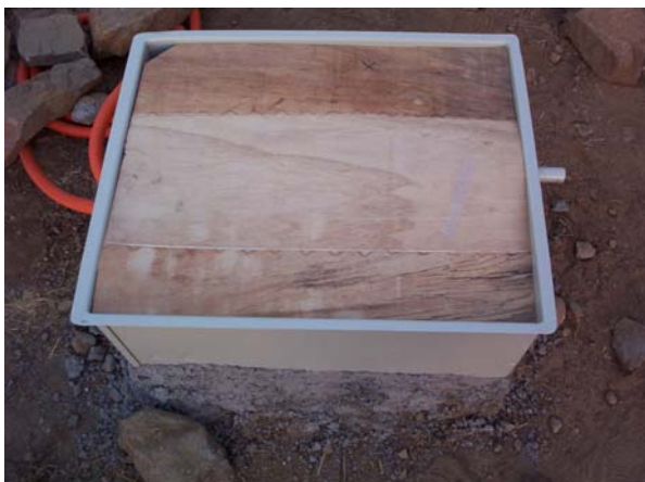
Metalic box to protect the receiver and batteries. Need a key to open the locker on the box.
