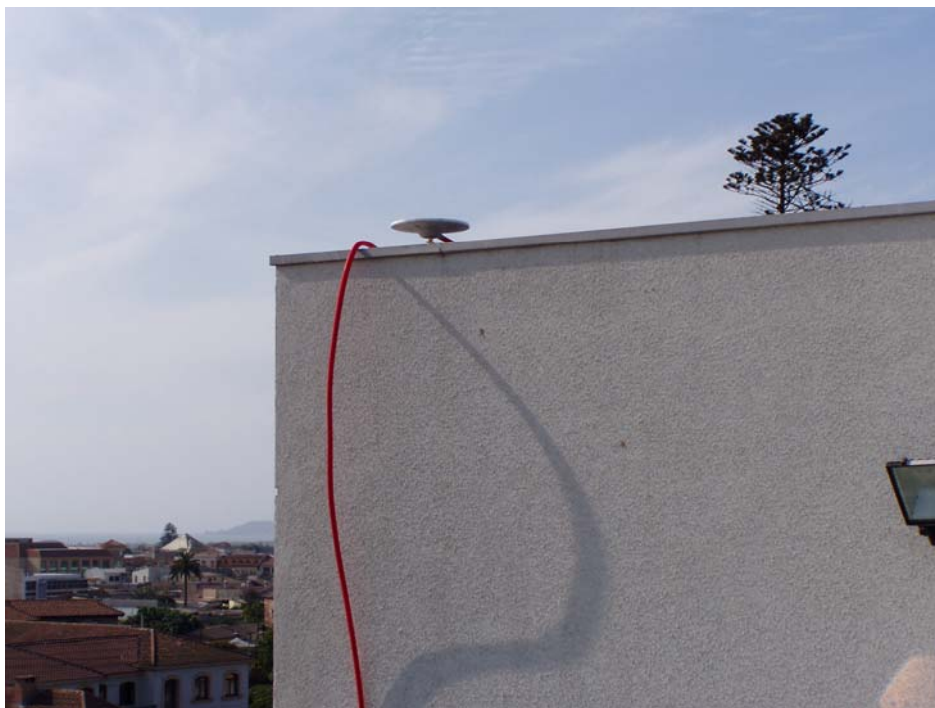
Antenna on the CETECFI Building roof.
