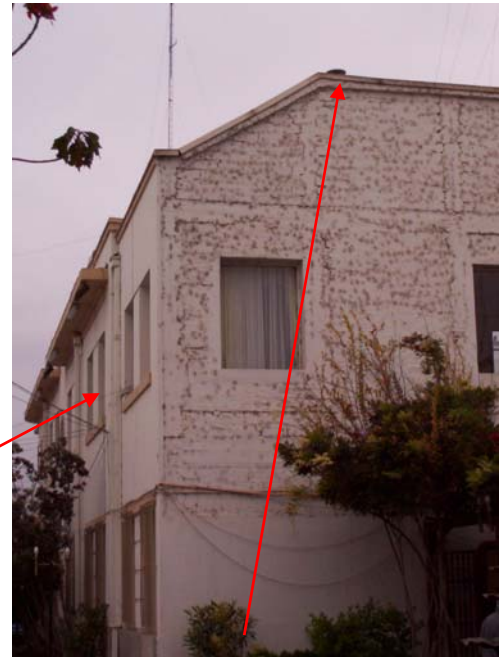
Antenna on the roof
