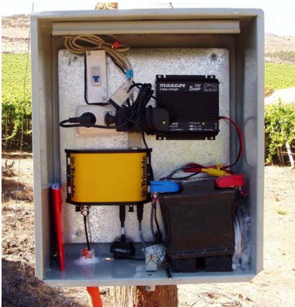
Installation in box with receiver, battery, charger and cables (220V power supply with 2A fuse)
