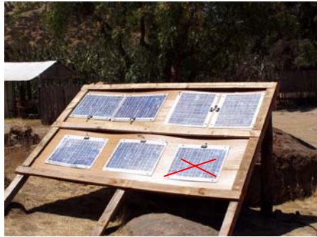
Solars pannels (6 since may 2007)
