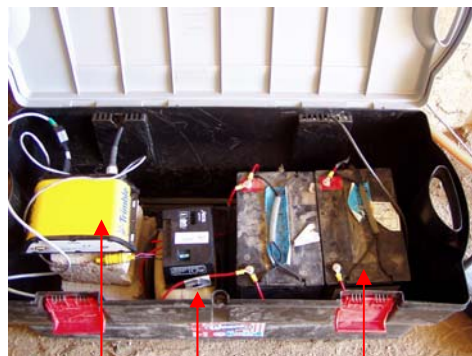
Receiver Regulator Batteries
