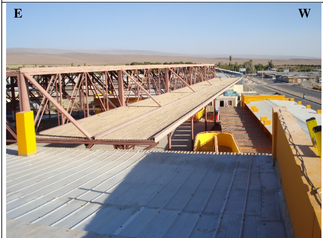
Photography N°4 : At SE of the antenna position is located a big metallic roof (made of iron) which top have the relative same level (height) than the antenna.
