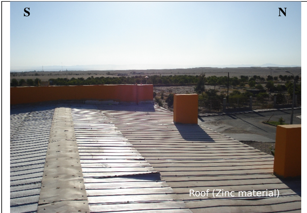
Photography N°3 :The roof of building is located directly to the east of the antenna
