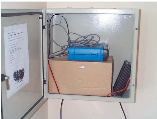
Upper left view : Cultural Center of the Mejikllones Municipality Upper right and central views : Geodetic GPS antenna on the top of the building Lower left view : metallic box with receptor Ashtech ZX and power supply
