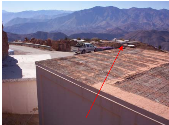
The antenna on the roof
